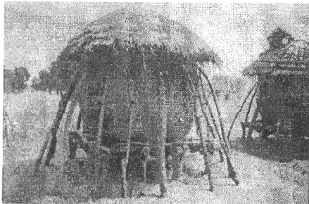
Plate 1a: Tree stem foundation assembly with supporting poles
